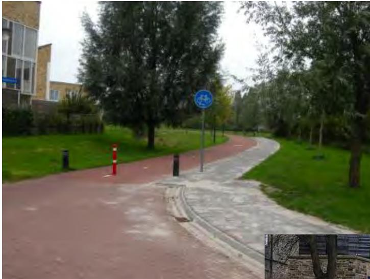
*A wide, two-way cycle path, with smooth surface, and lack of obstacles on entry. Cycle paths like this should serve as shortcuts, routes that are not available to motor vehicles. Note also a clearly demarcated pavement, which should be present where pedestrian and cycle movements are high, as is typical throughout London, to prevent conflict. This example is from a new development in Assen, the Netherlands.*
