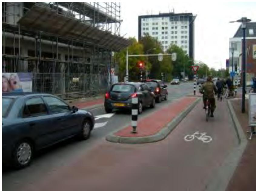
*Dutch minor signal-controlled junction, in Assen. Motorists and cyclists move through the junction in separate phases*
