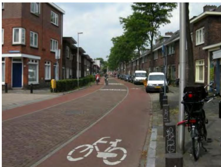
*In this example, from Utrecht, NL, space for cycle lanes of adequate width is achieved through making the street one-way for motor vehicles*
