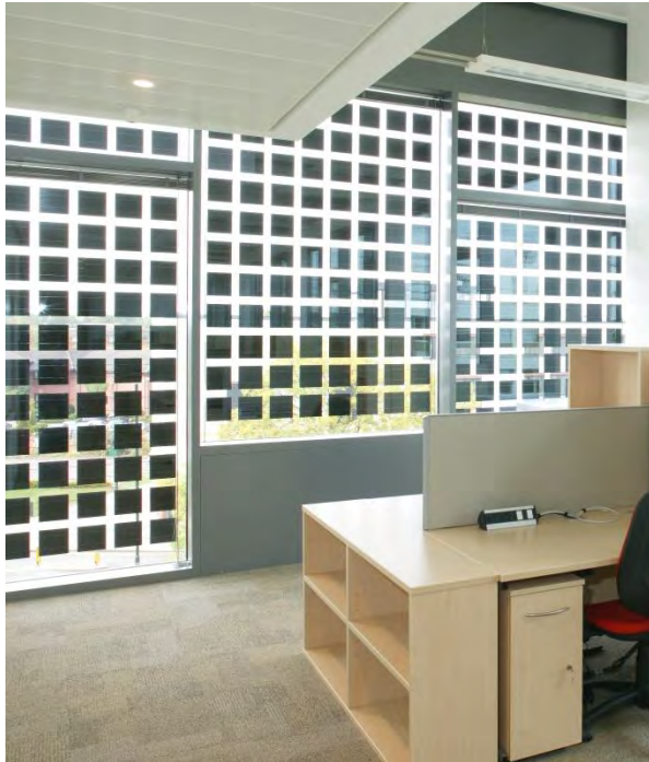
Figure 8. CPW Solar Glazing Installation, University of Warwick - Materials and Analytical Sciences Building
