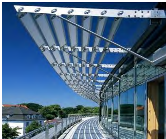
Figure 7. Solar PV Louvres on the South Facade
