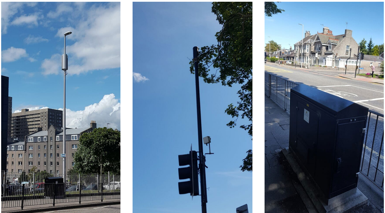
Figure 6 – Wireless Infrastructure Provider WIG have installed a neutral host network on a main road in Aberdeen. Mobile operator equipment is housed in standard green cabinets adjacent to street furniture
