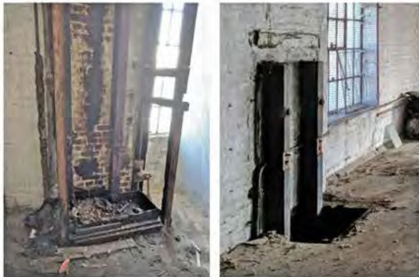
Figure 32. HOIST TYPE 1 – Modern hydraulic hoist machinery & timber casing to second floor lost.
