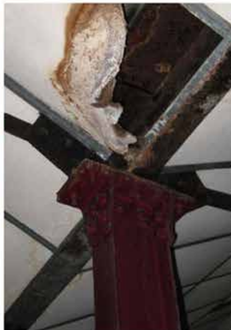
Fig. 41: Detail view of the head of a typical 3 rd floor steel column supporting the roof trusses and valley gutter
