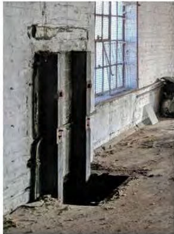
Figure 33. HOIST TYPE 1 – Modern hydraulic hoist machinery & timber casing to third floor lost.
