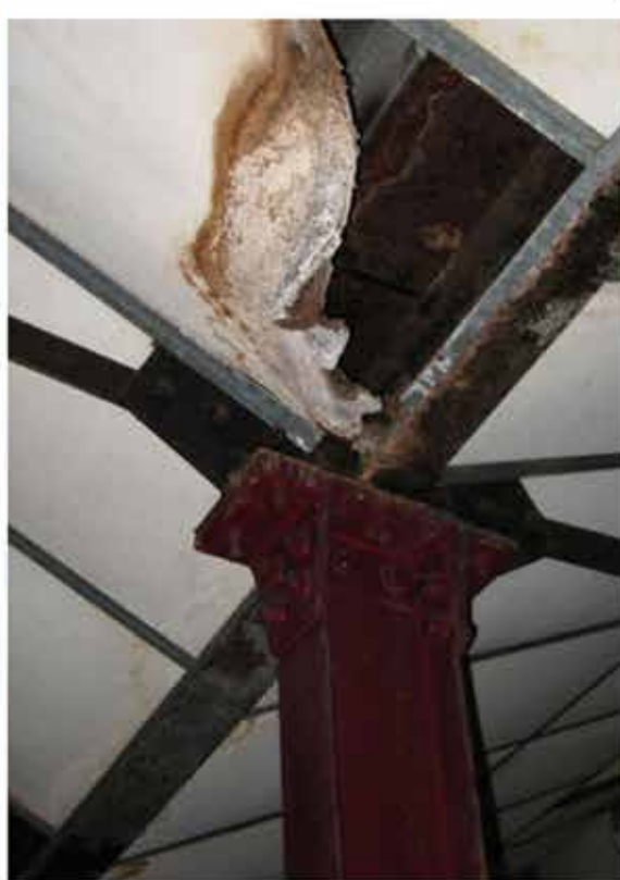
Figure 13. COLUMN TYPE 2 – 1940s rolled steel column to Third floor, supporting steel trussed.
