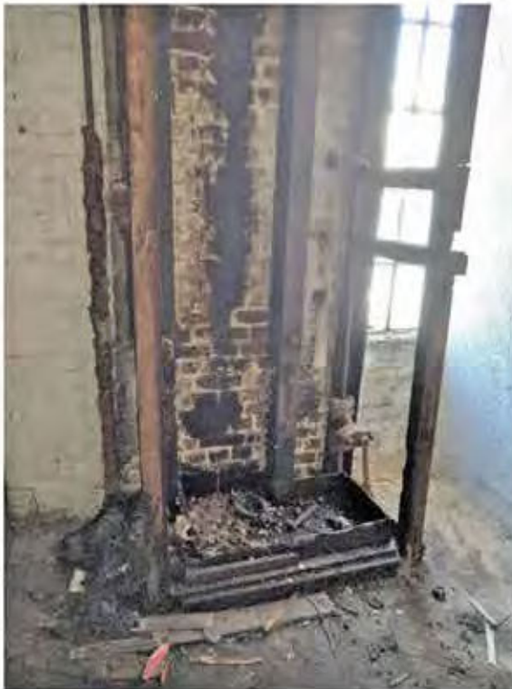
Figure 32. HOIST TYPE 1 – Modern hydraulic hoist machinery & timber casing to second floor lost.
