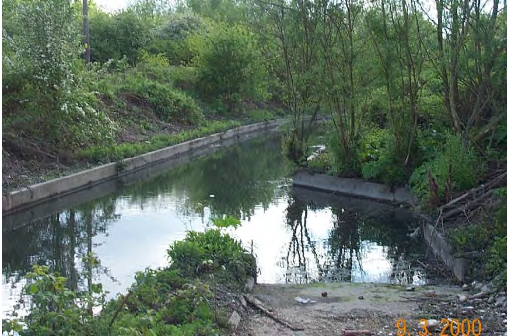
Photo 1 Flood Relief Channel
