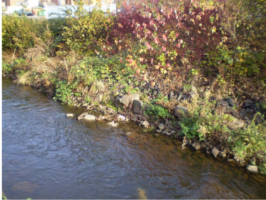
Photo 3 River Stour, Kidderminster Naturalised Rock Armour
