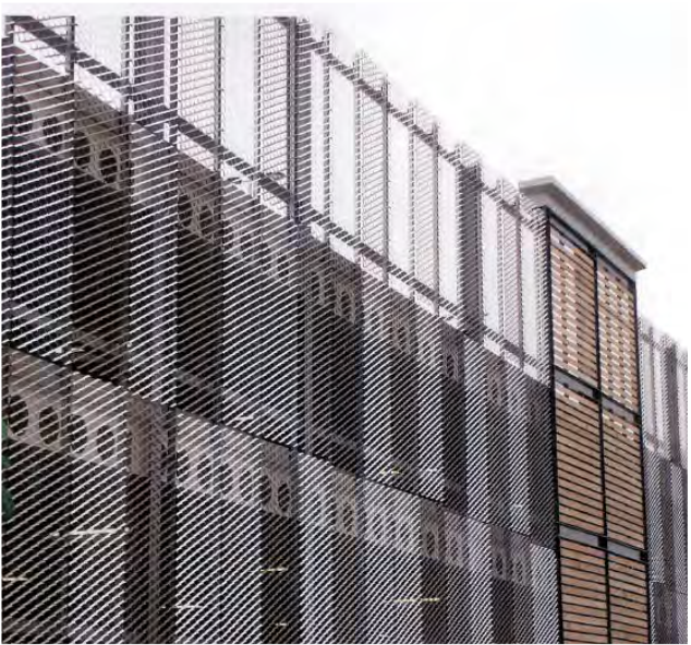
Illustrative elevation demonstrating perforated anodized finished aluminium panels
