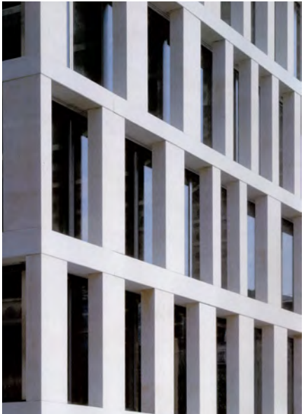
Illustrative elevation demonstrating cast natural stone
