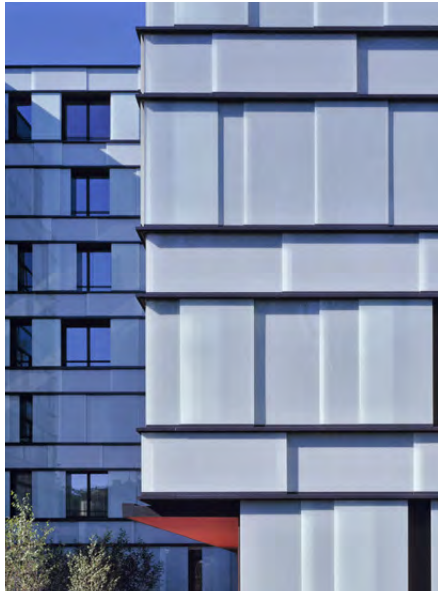
Illustrative elevation demonstrating opaque glass
