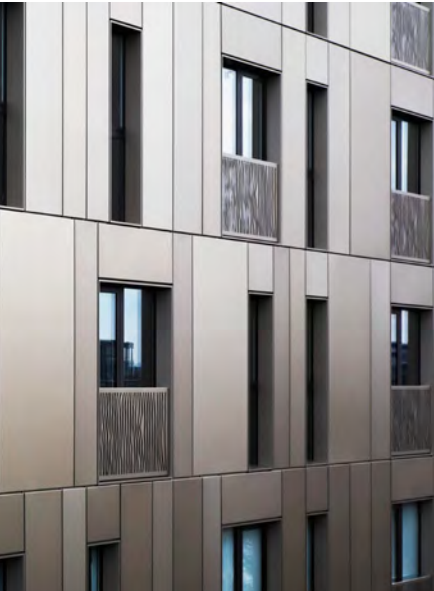
Illustrative elevation demonstrating anodised aluminium panels
