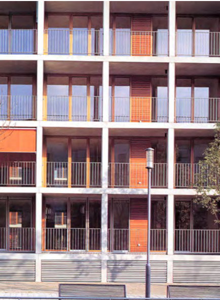
Illustrative elevation demonstrating cast stone exposed structure
