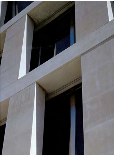
Illustrative elevation demonstrating cast natural stone
