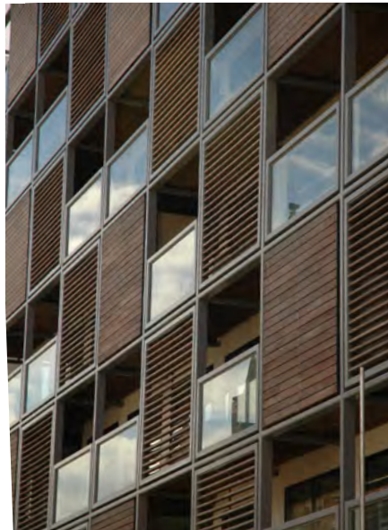
Illustrative elevation demonstrating hardwood and glass balconies
