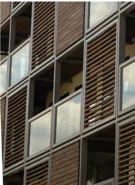
Illustrative elevation demonstrating hardwood and glass balustrades
