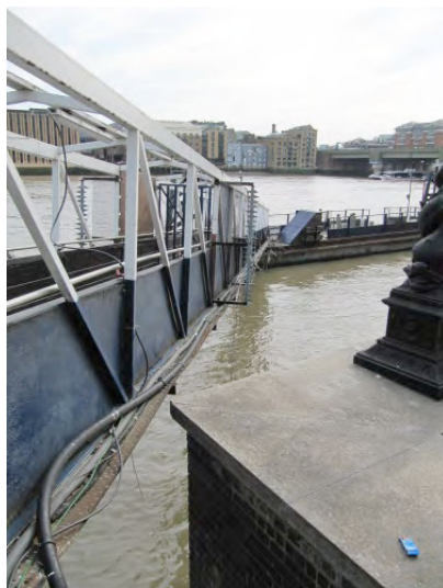
Figure 2: Services on an existing pontoon bridge in the Thames
