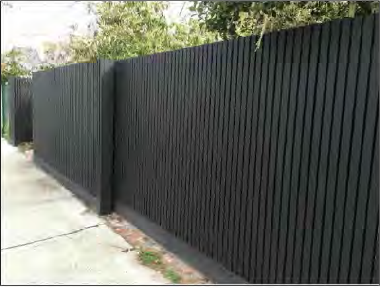
Timber acoustic fence
