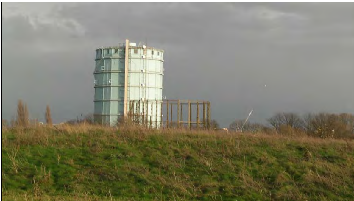
Figure 16.3 The box-lattice standards of No. 3 in front of the ‘blue tower’ fixed gasholder (be retained).
