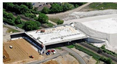
**Purpose of assessment** To compare embodied carbon footprint for the use of expanded clay and EPS (expanded polystyrene) against a granular aggregate benchmark (6N) in the backfill section of Cottingham Road overbridge.
