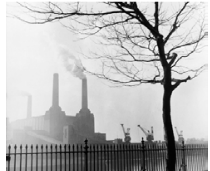
BATTERSEA POWER STATION, 1950 –1959 © Henry Grant Collection/Museum of London
