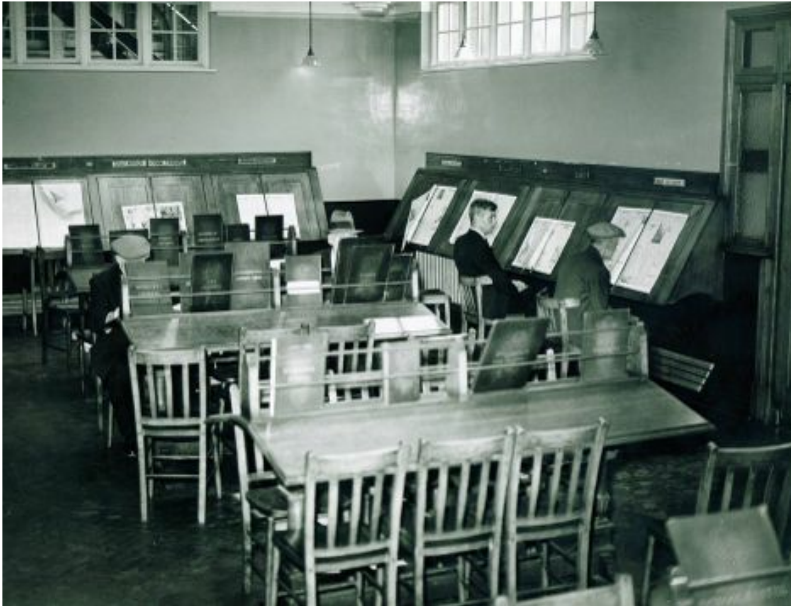
Manor Park Library Newspaper Room, at rear extension The room features highly specific bespoke furniture
