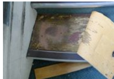
Floors stairs and landing
