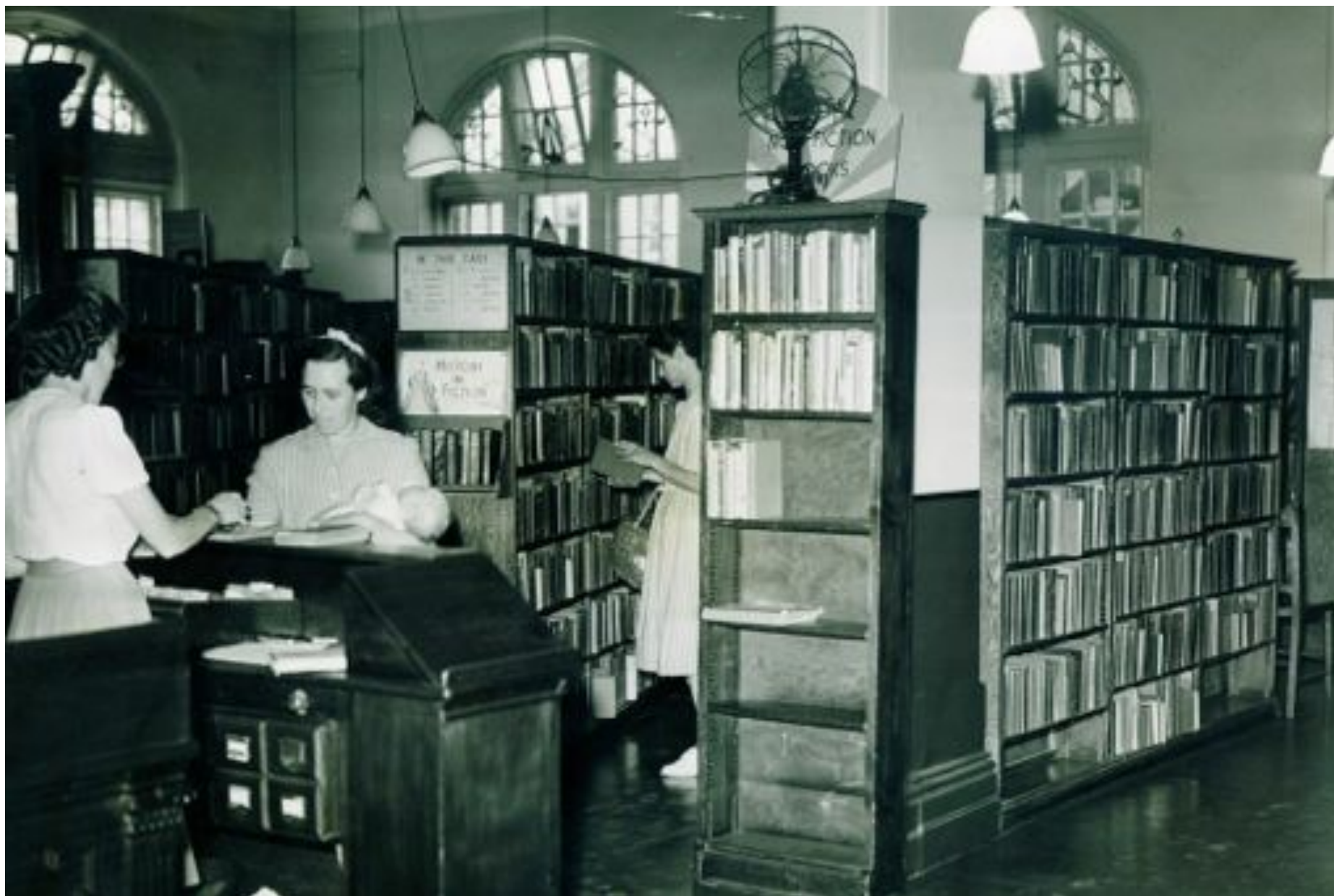
Manor Park Library Stack Room with radiating shelves, 1946 Note that in the photo that there was only one column
