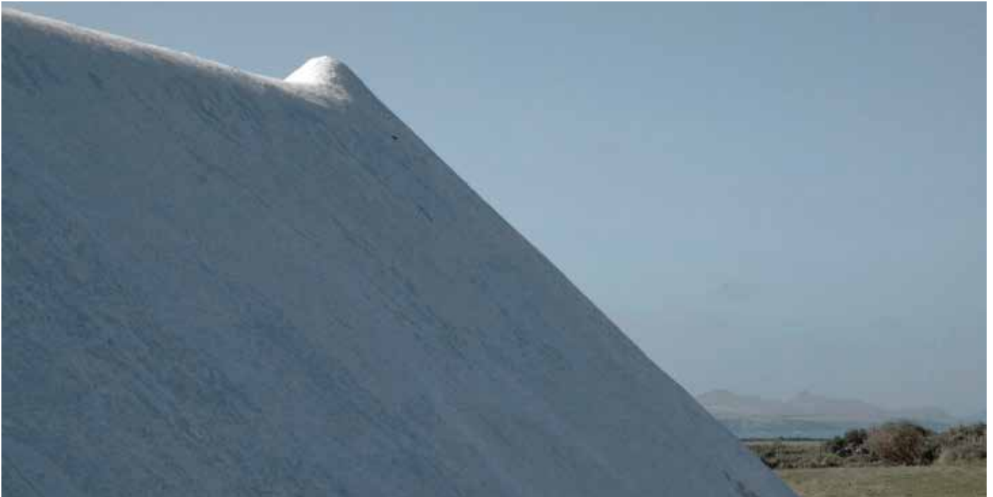
Traditional grouted roof
