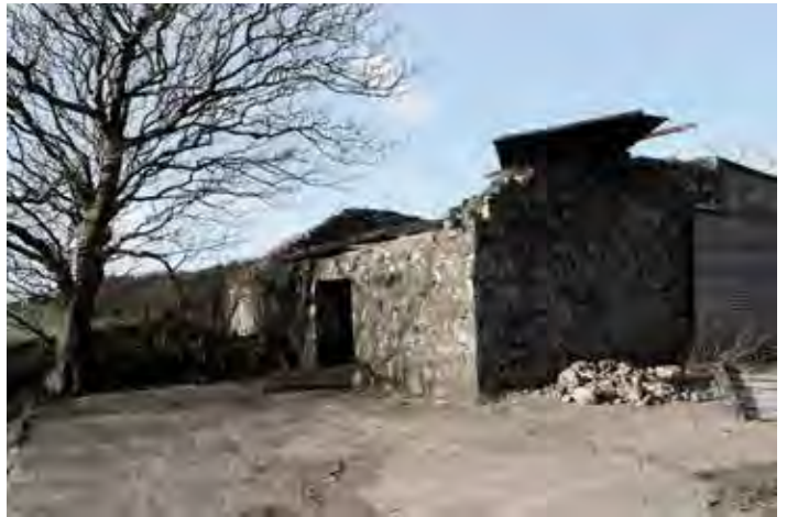
Ruined cottage before restoration
