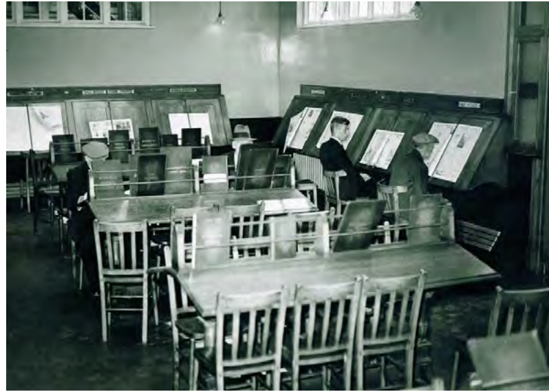
Manor Park Library Newspaper Room, at rear extension The room features highly specific bespoke furniture
