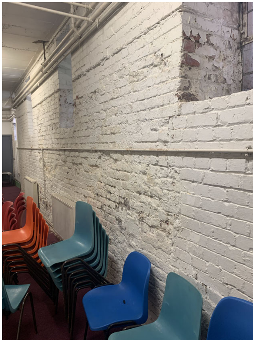
Image 3: View towards the left of the northwest basement wall, showing original and refurbished brickwork
