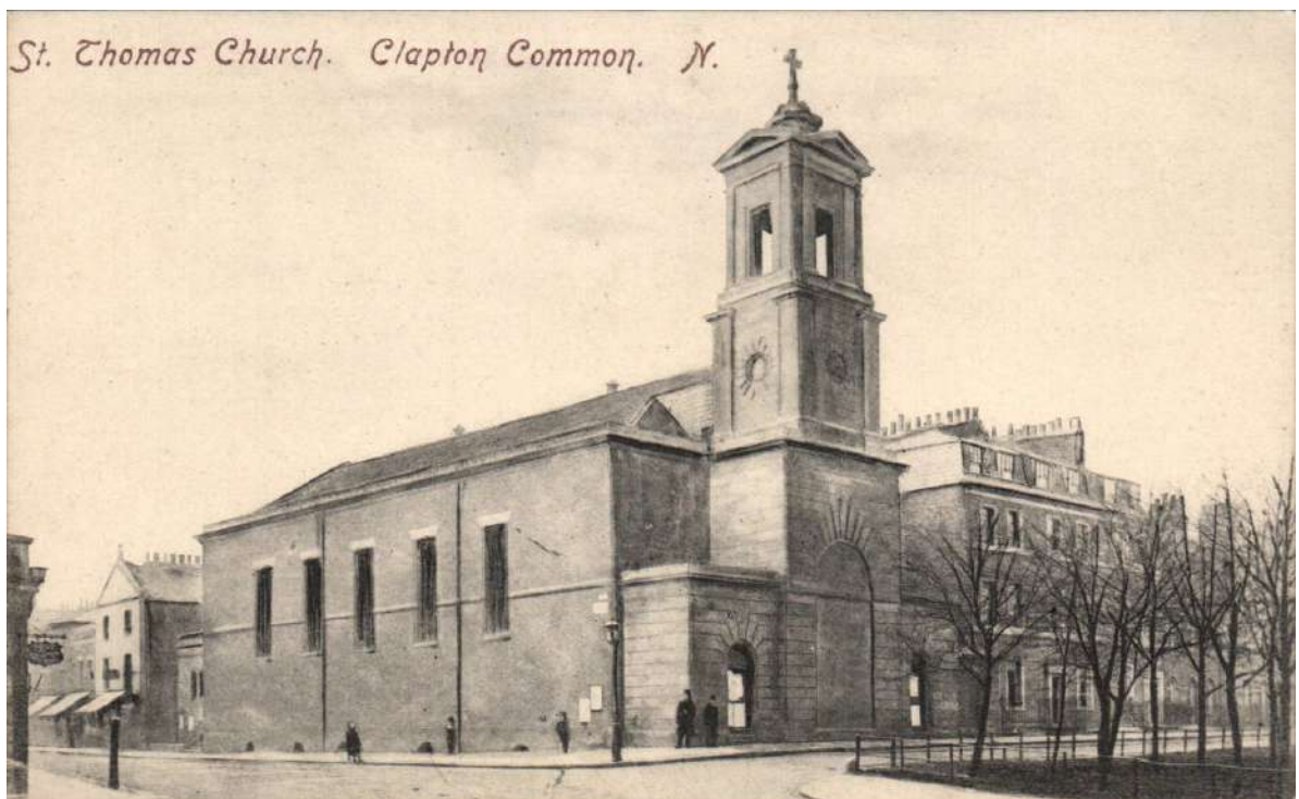
View from the east side showing the original nave, with Joseph Gwilt's tower and porches added in 1828.
