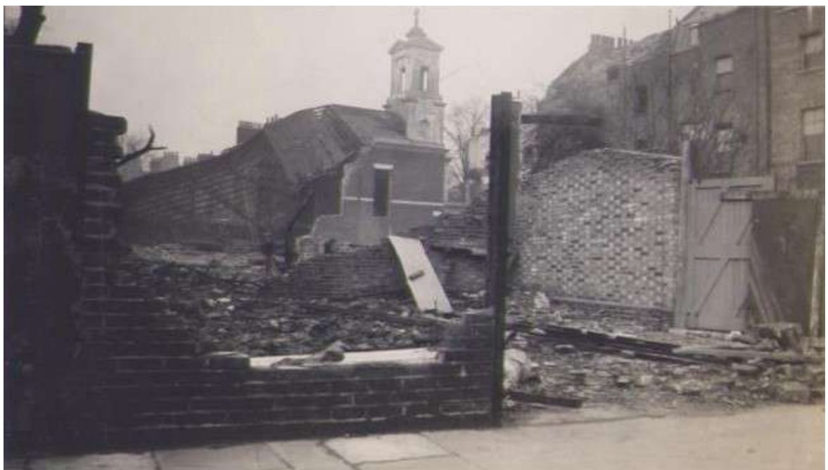
1940 bomb damage to the nave, viewed from the south, showing the tower remaining.
