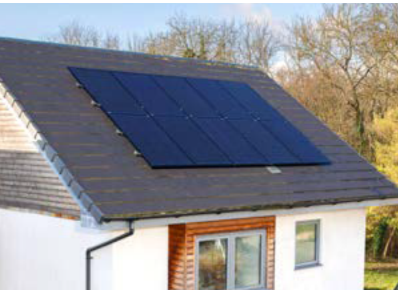
IKEA: Solar Panels
