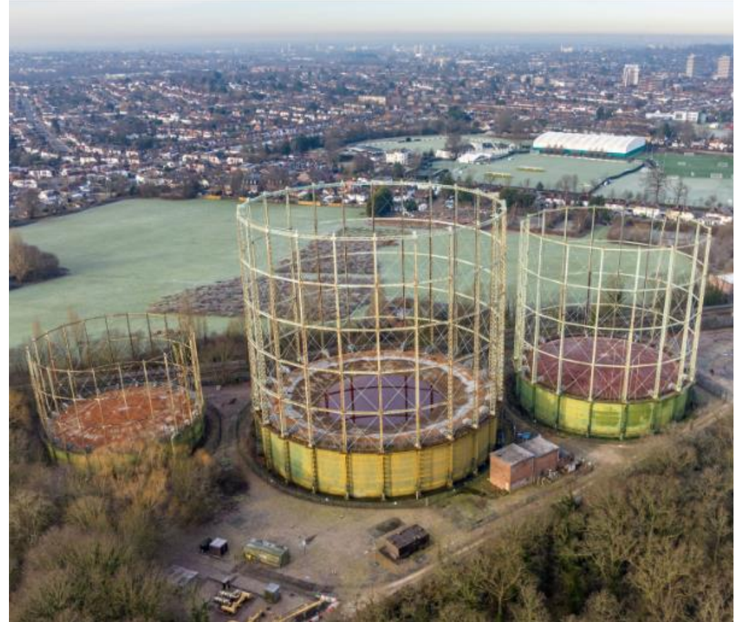
Heights of Gasholders 26m, 59m, 49m
