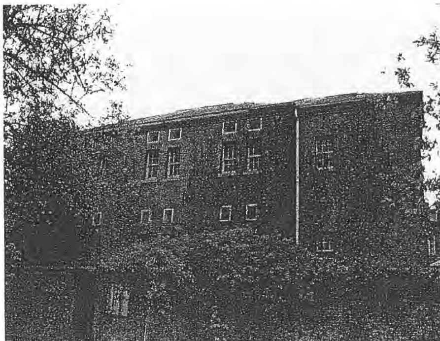
02 NW elevation and lean-to structure
