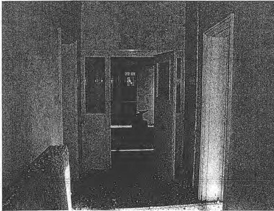
09 Second floor corridor - north end
