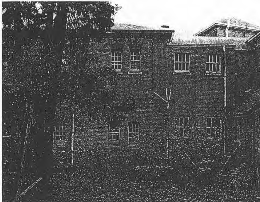
04 W. elevation of rear addition of 16B
