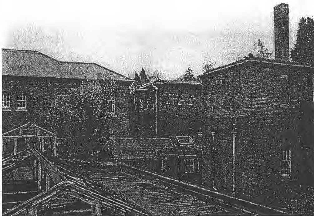
03 South elevation to west & east blocks
