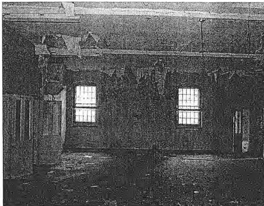
05 Condition within 14A
