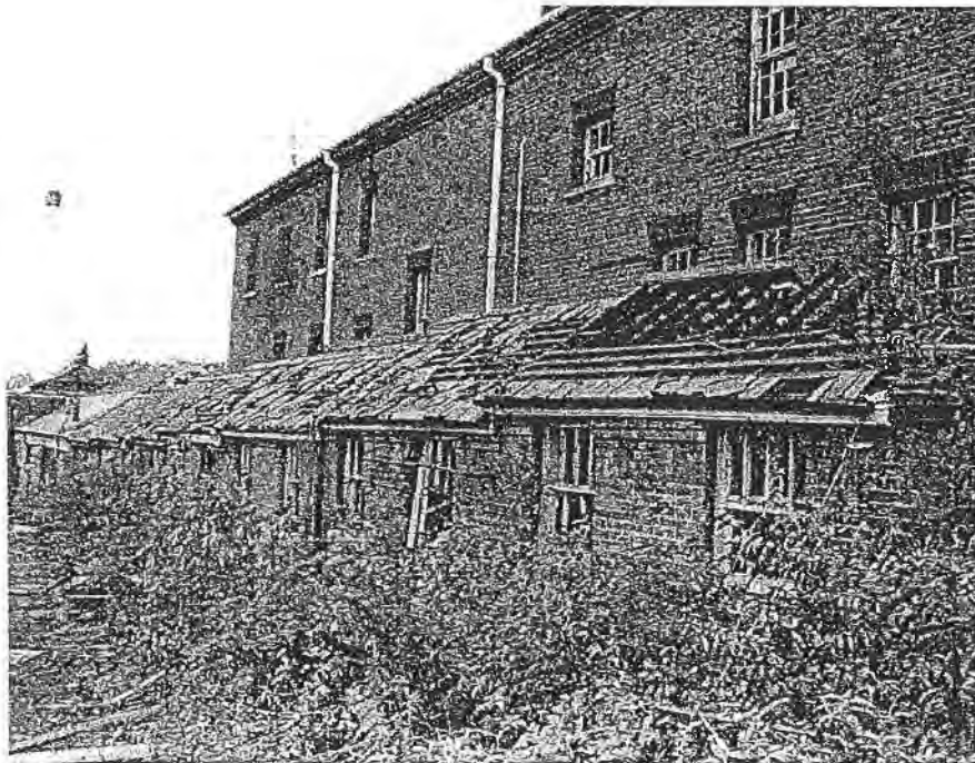
02 SW Elevation of 14A
