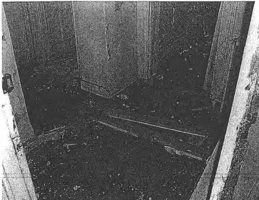
05. Collapsed floor
