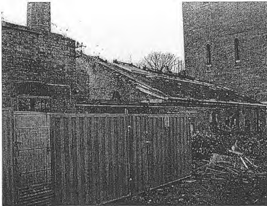
03 NE Elevation of 14B
