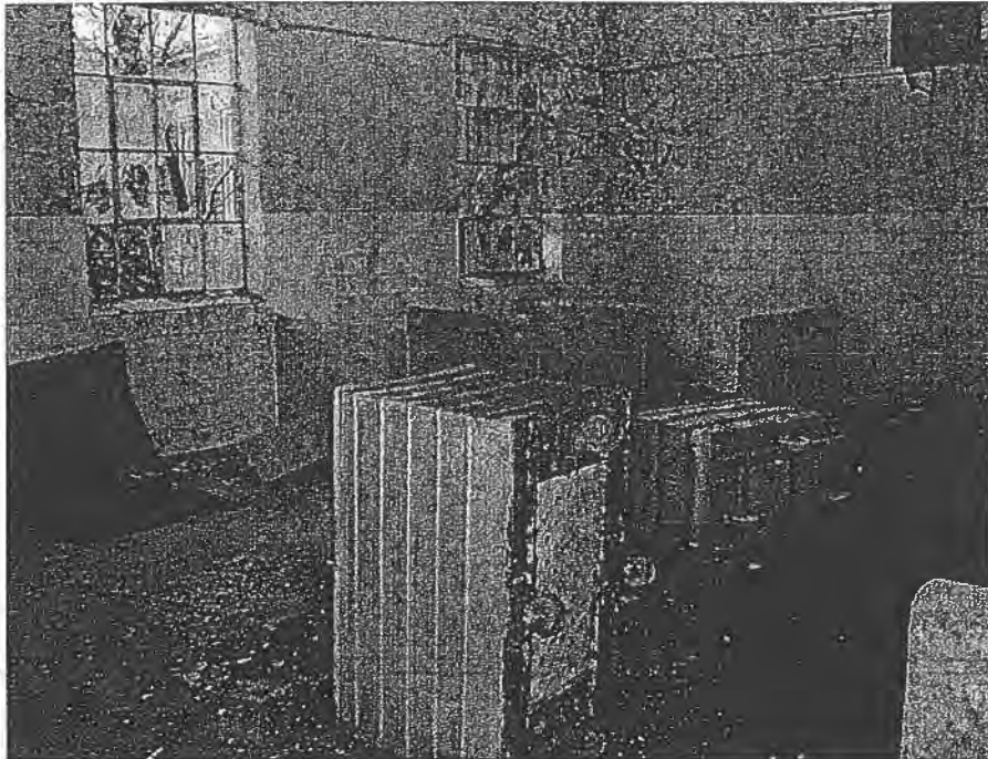
07 Typical conditions of rooms in 13A
