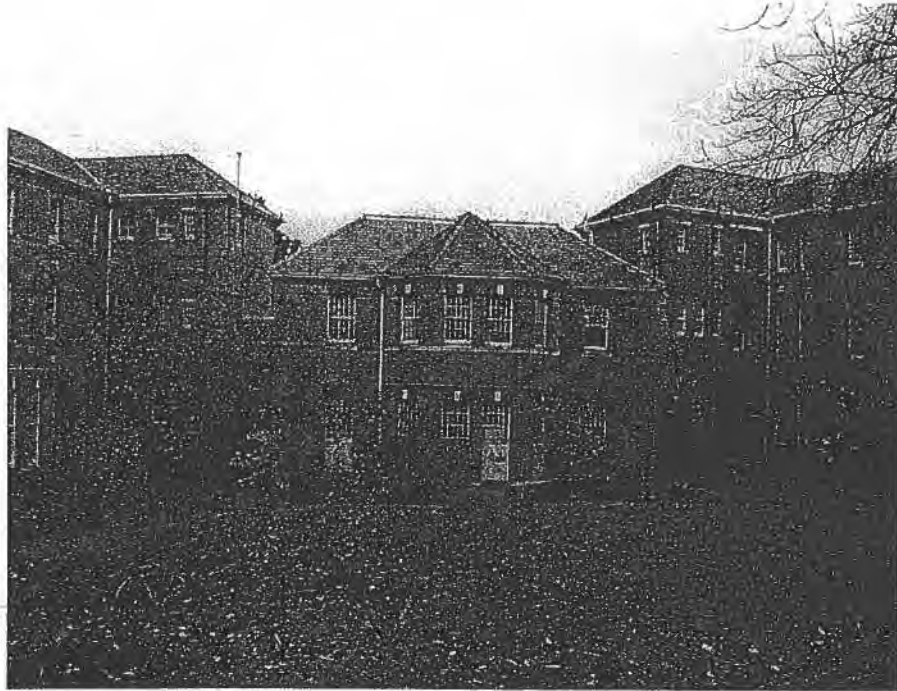
03 South elevation of 16B
