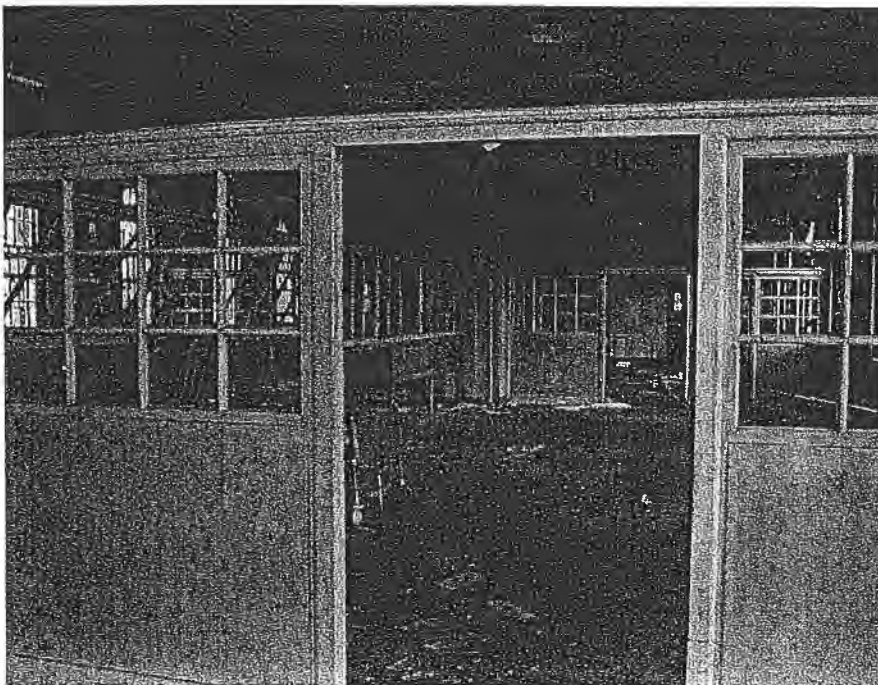
06 1st floor dormitory
