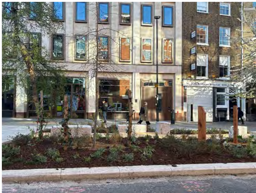
Figure 34: Rain garden retrofit in a central reservation at St John Street, Islington
