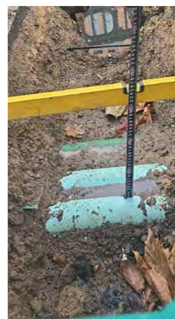
Figure 15: Trial holes
