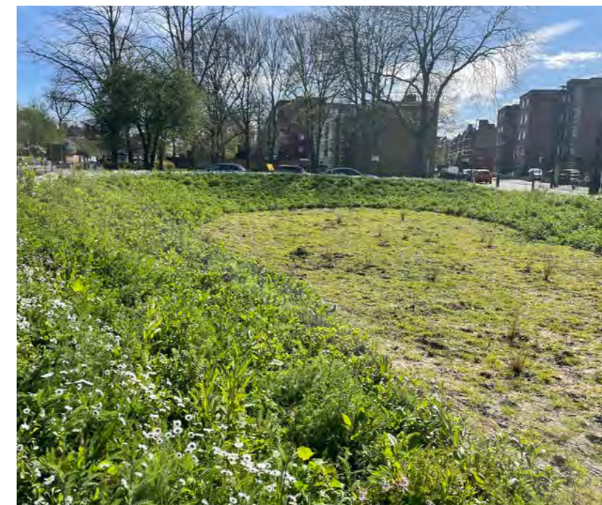
Figure 6: Swale retrofit at St Matthew's Estate, Lambeth
