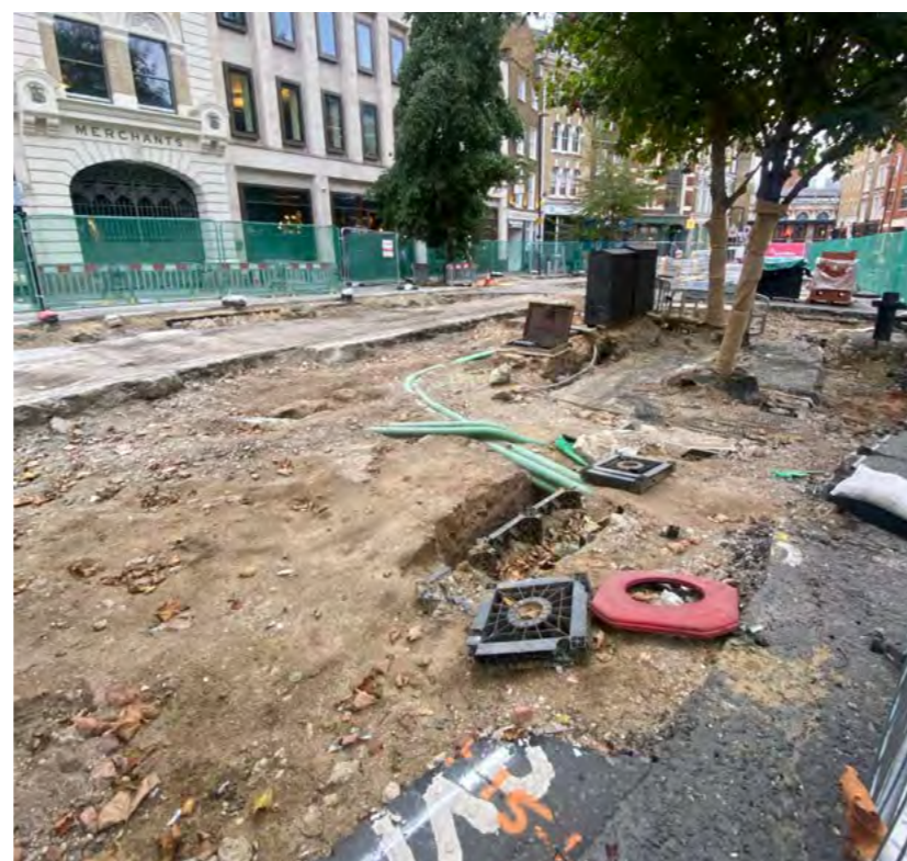
Figure 51: Rain garden retrofit in a central reservation at St John Street, Islington
