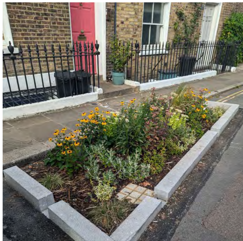
Figure 29: Rain garden retrofit in a build out at Charlton Place, Islington
