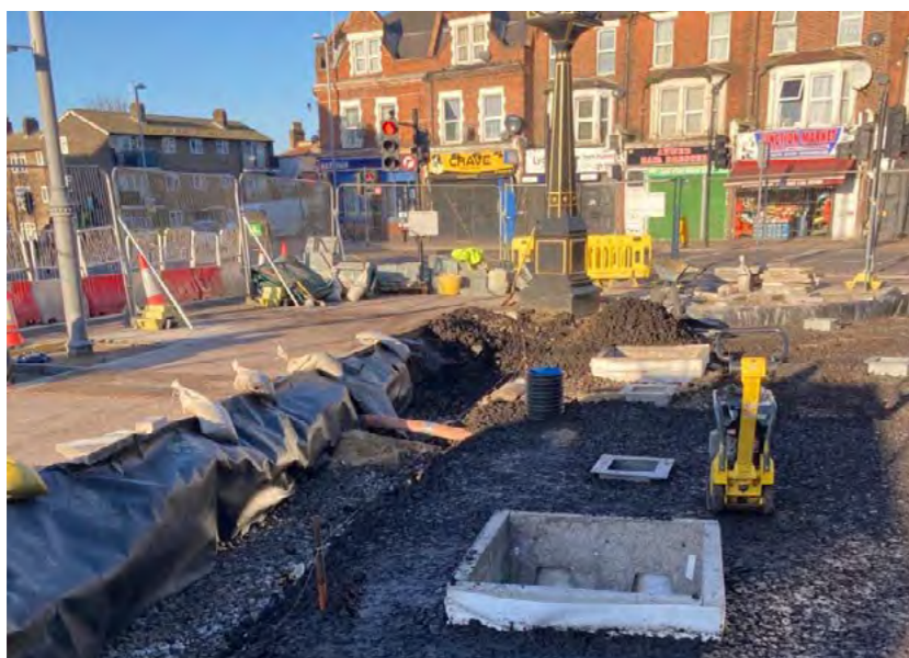
Figure 46: Structural Soils being implemented at Markhouse Corner, London Borough of Waltham Forest
