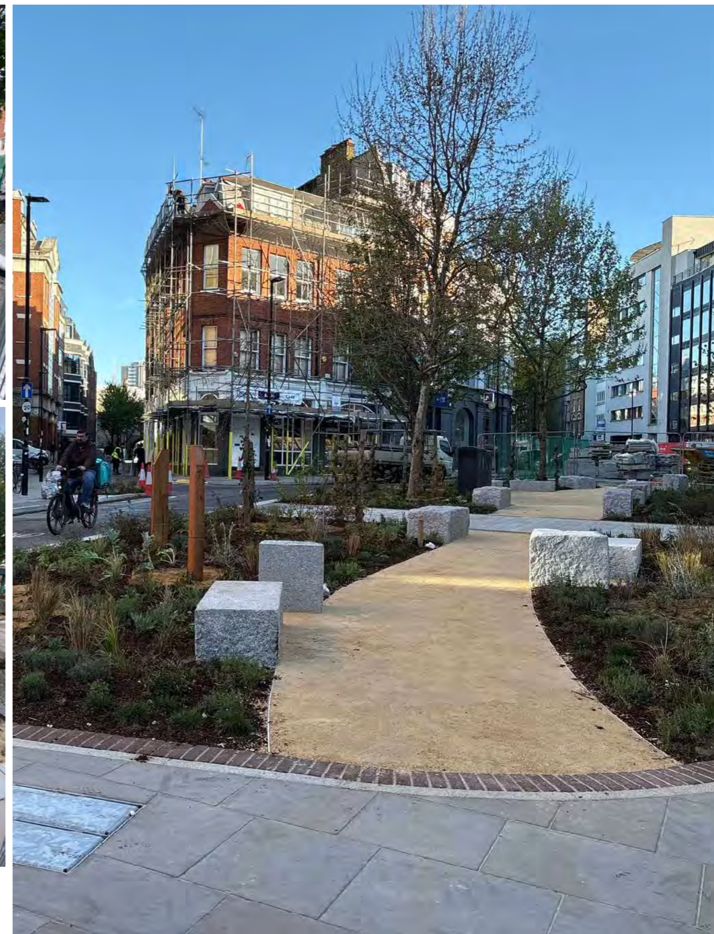
Figure 55: Completed scheme at St John Street [credit: Meristem Design]
