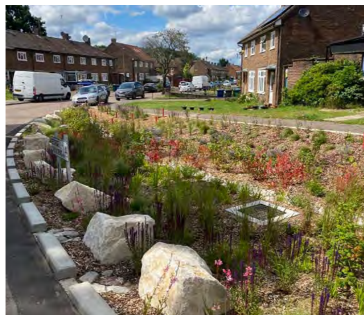
Figure 37: After photo, retrofitted with rain garden - George Crescent, Barnet [credit: Meristem Design]
