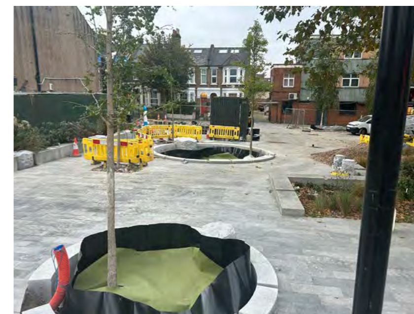
Figure 16: Construction underway at Juniper Pocket Park
