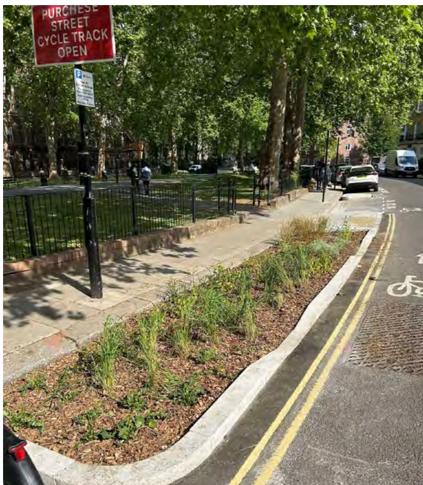
Figure 21: low-growing planting chosen for rain garden at Somers Town, Camden [credit: Meristem Design]
