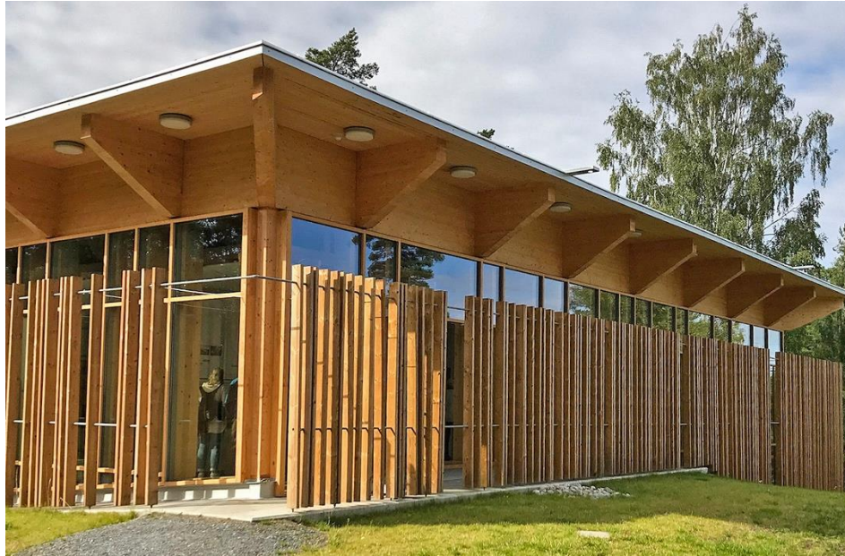
The “Hegnhuset” building on the island of Utøya covers the original café building. (Photo: Kjell Brataas)
