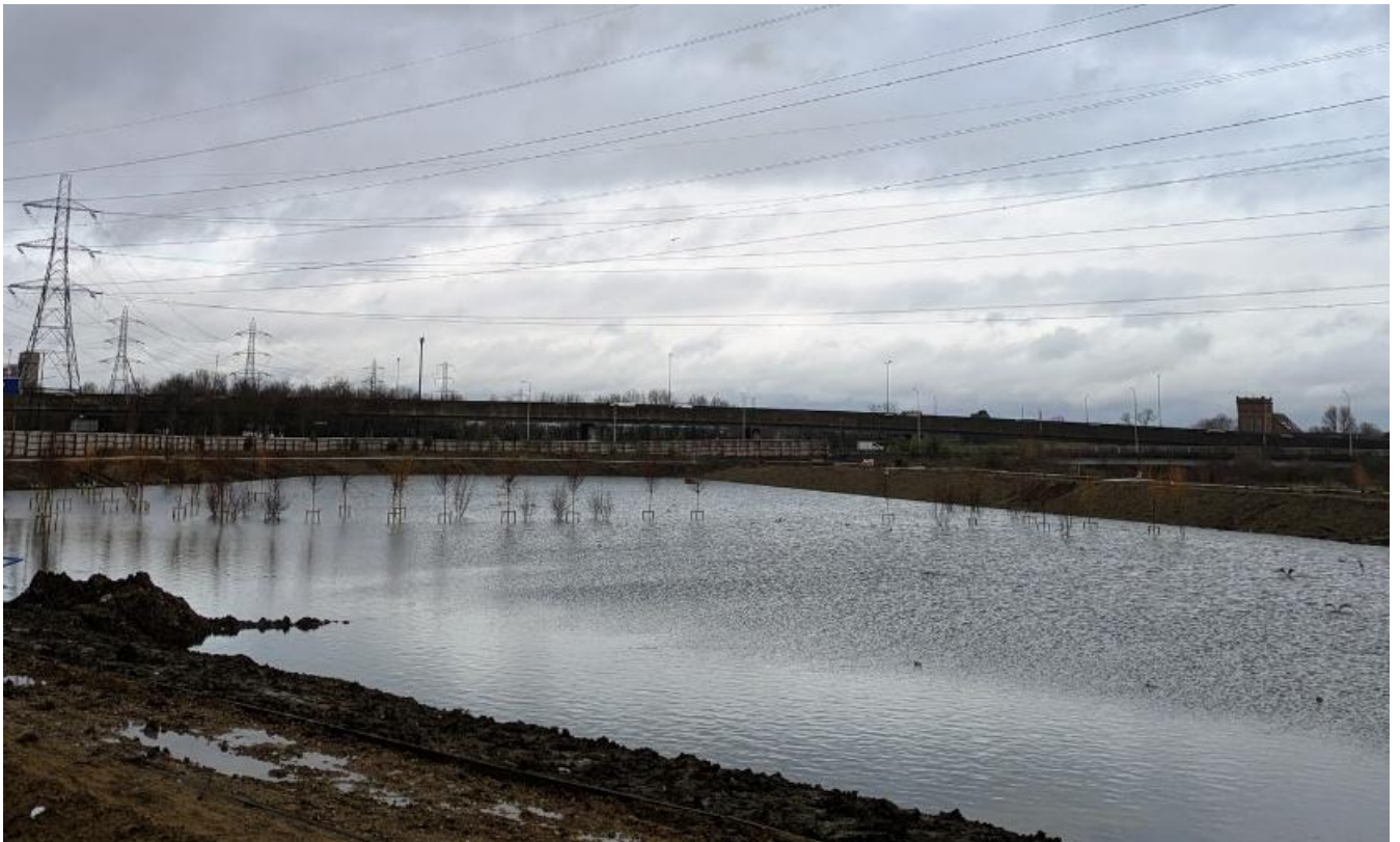
Figure 25 - A new park in southeast Enfield at Meridian Water has been routinely flooded (it is the new settlements main park but its utility as a function public park will be limited during wet weather months)
