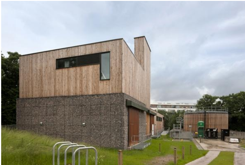
Figure 24 - Old Ford Water Recycling Plant - Source: Architects' Journal (2012)
