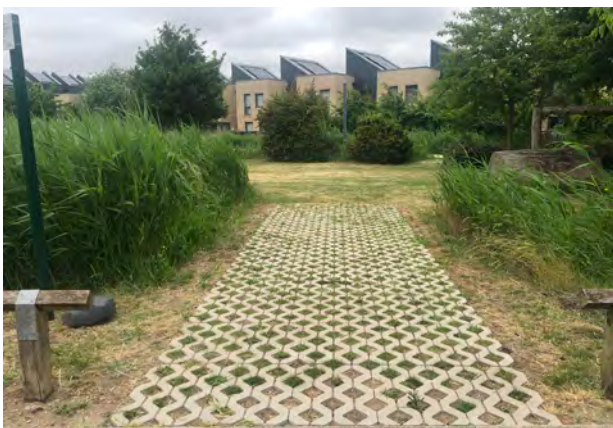
Permeable paving and other SUDS in Barking (including swales) are attractively integrated into the open space network
