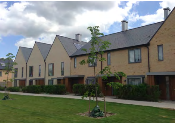
Two storey terraced homes create a compact urban form, increasing density and maximising land efficiency
