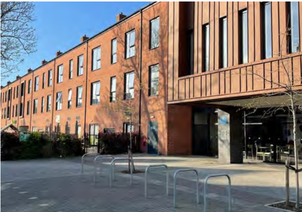
Apartments alongside non-residential uses bring activity to the heart of the development in Manchester
