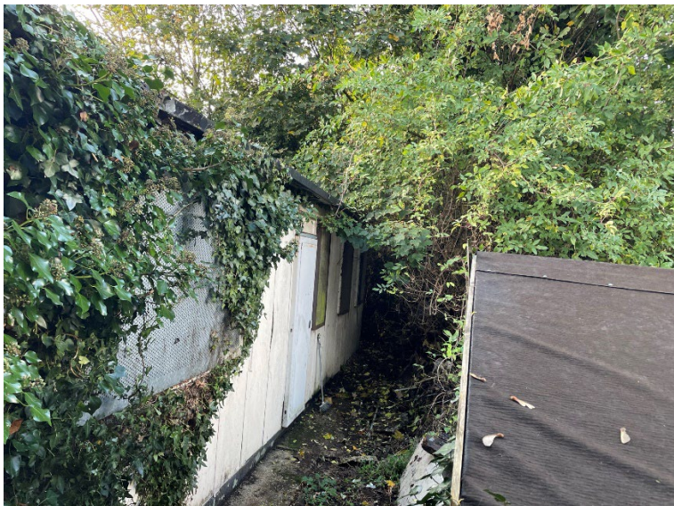
Above: Image of existing structure on the site
