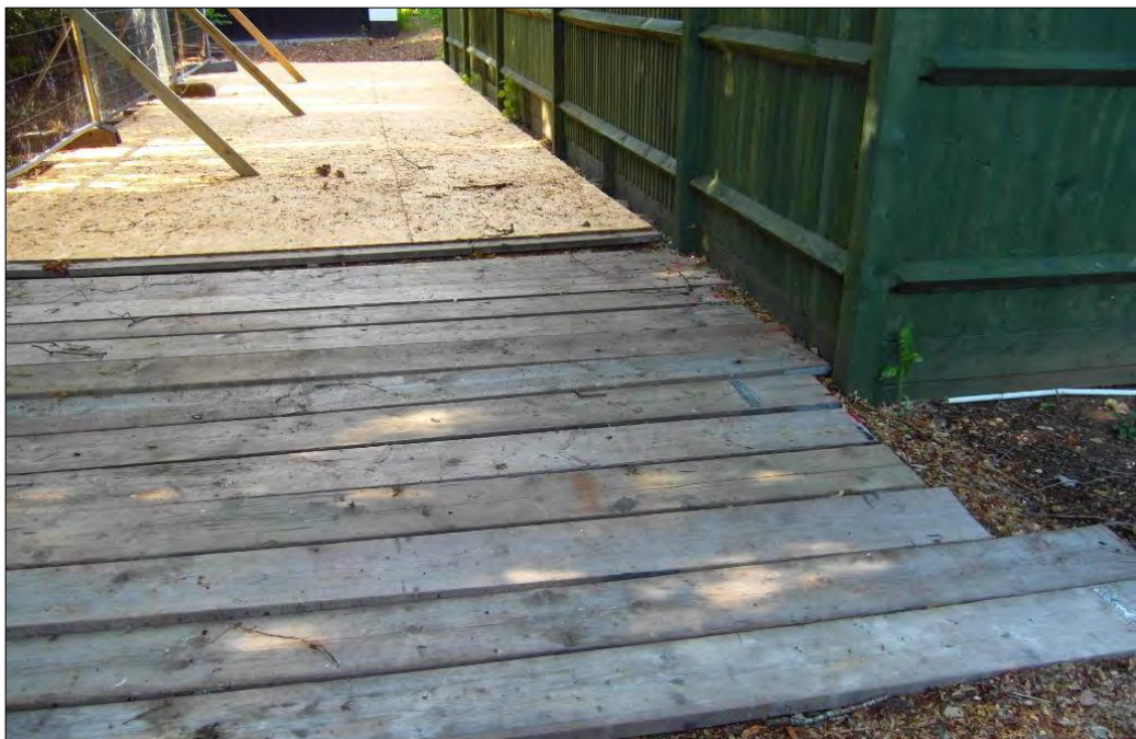
Fig.2 Side-butting scaffold boards and covered and fixed with 20mm OSB boarding
