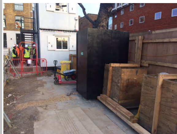
Robust hoarding and temporary concrete ground protection
