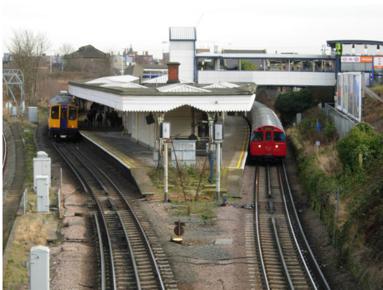
Fig.32. Willesden Junction station
