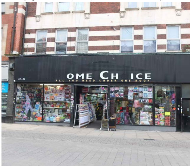
Fig.29. Shop front in the High Street
