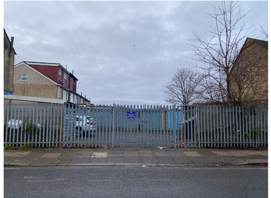
External front view of the site
