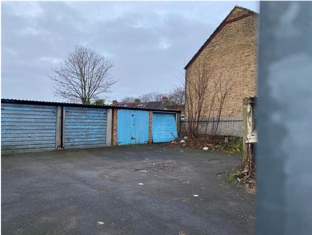
Internal view of the site showing four of the garages
