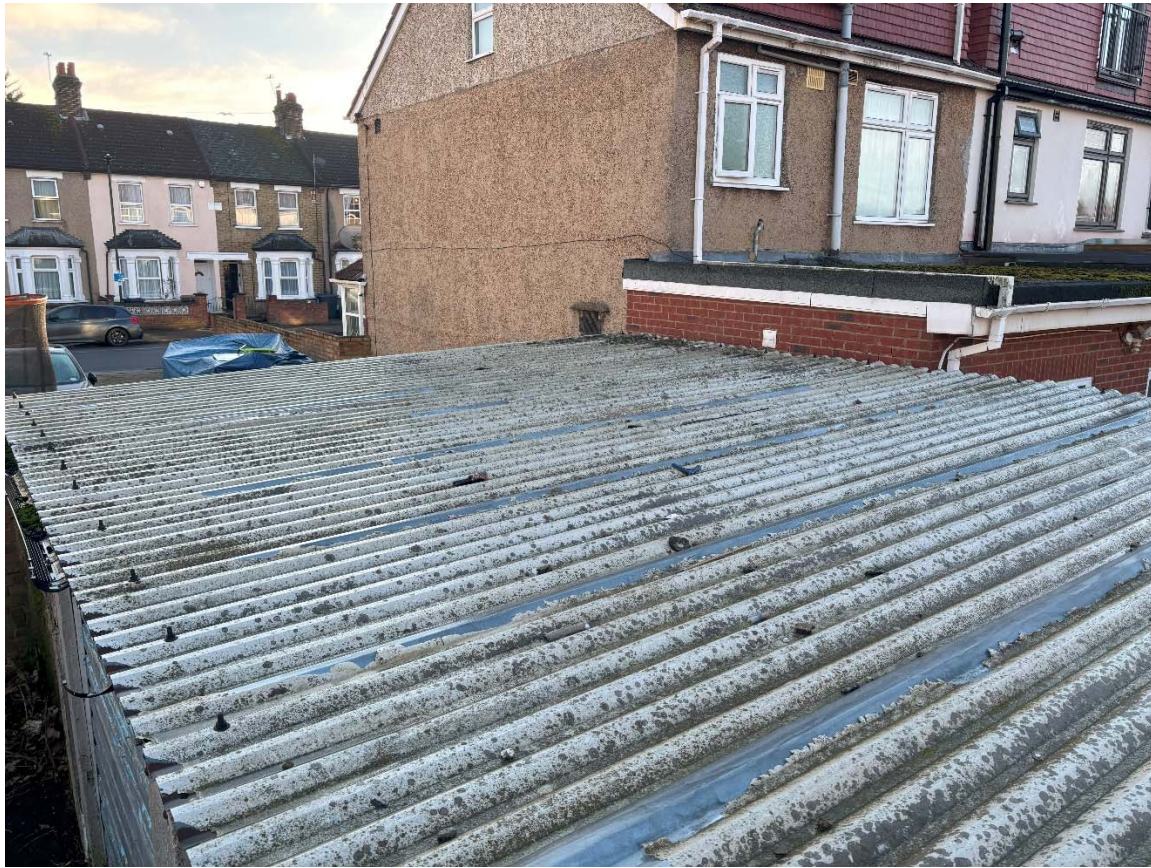
Image 3 – Flank wall of 114 Regina Road (NB: extractor louvre in extension wall)
