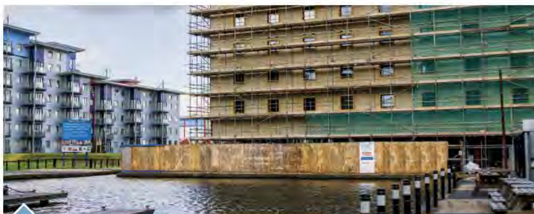
Premier Inn, Walsall Waterfront: 9mm Y-wall is used as the fire rated sheathing board, total quantity used 1,800m 2 .
