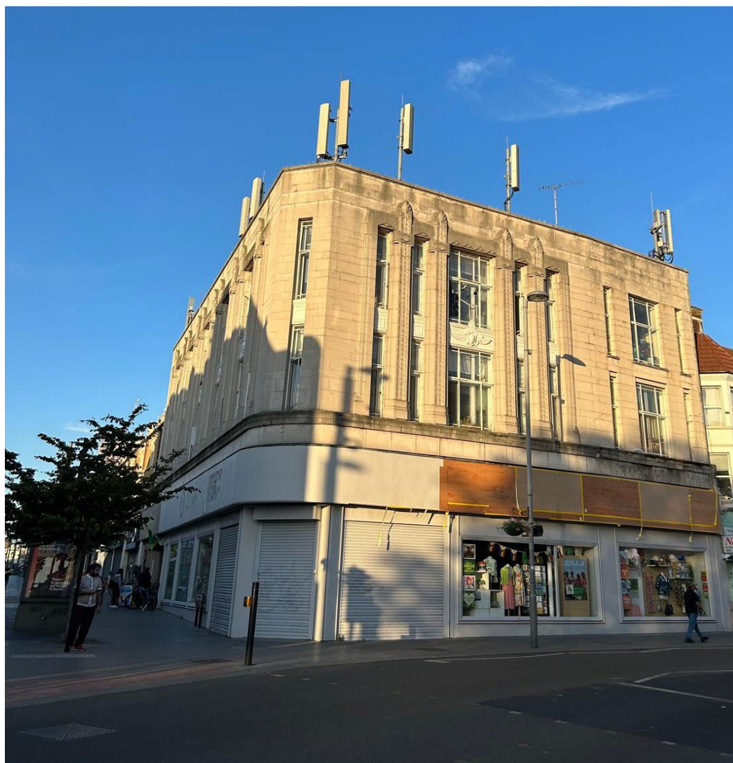
Figure 2.1 Building within a conservation area with poorly located DCI that is highly visible and dominates the building roofline.
