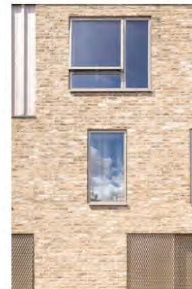
✓ Fig. 160. Coherent use of brickwork across a facade. London
