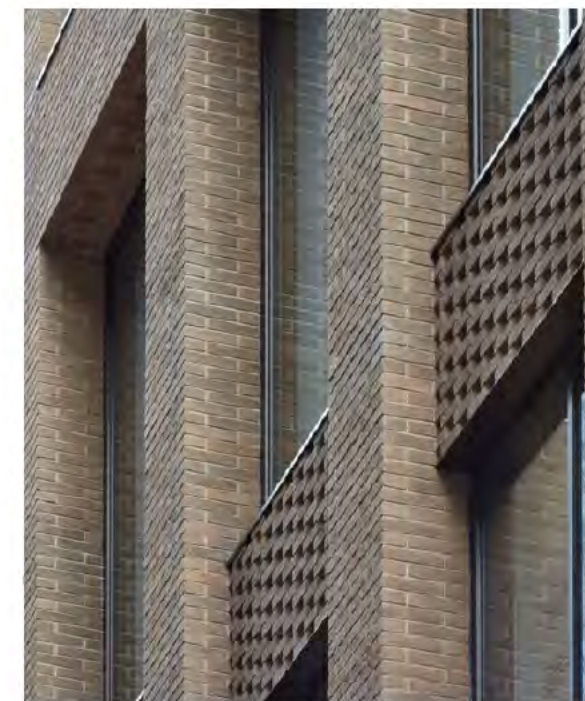
✓ Fig. 161. Depth added to the facade using 'hit and miss' brick coursing. London
