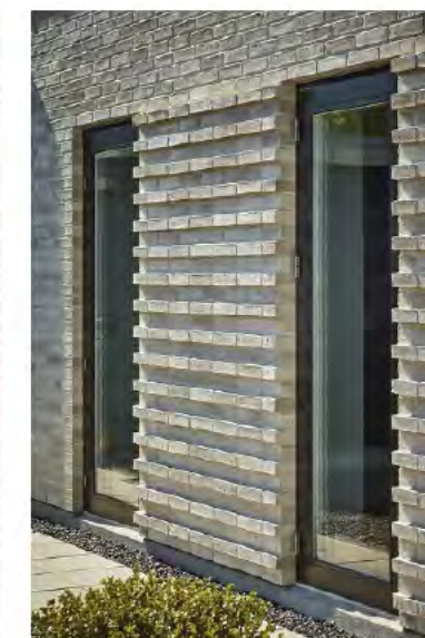
✓ Fig. 162. High quality detailed brickwork. Silchester Estate, London
