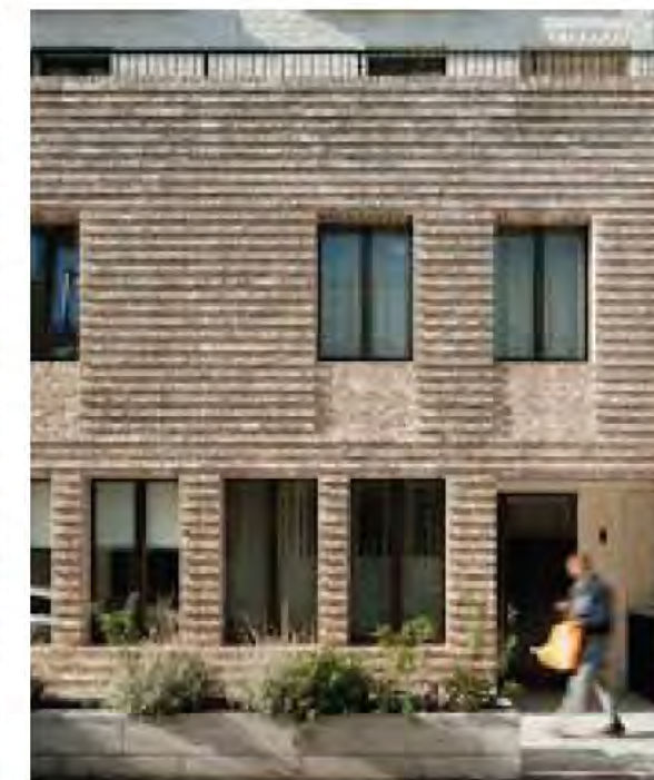
✓ Fig. 164. Texture is added to the facade by subtle changes in brickwork around windows. Silchester Estate, London
