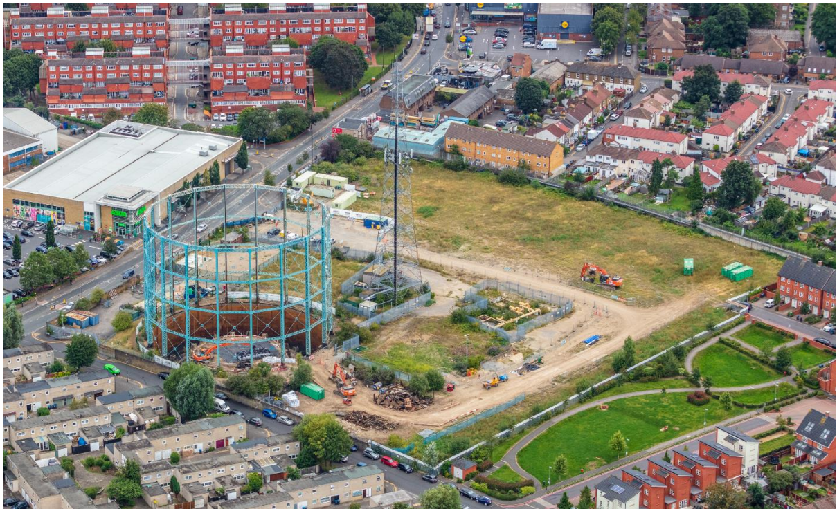
Aerial view looking east during gasholder demolition. One PRS can be seen in the centre of the site, with another behind the gasholder. Telecoms mast is in the centre of the site - 2021
