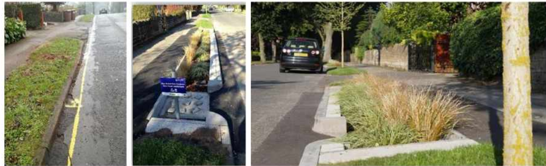
Figure 5.13 Greening streets, retrofit rain gardens at SuDS Project in Ribblesdale Road, Sherwood (before and after)
