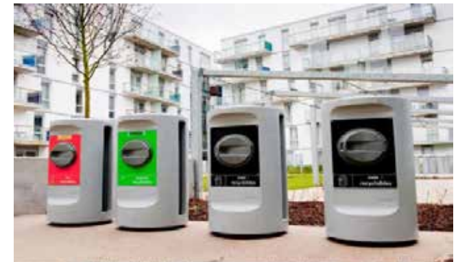
Figure 5.5. Pneumatic waste collection system
