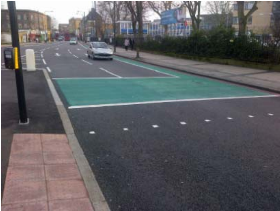
Newly constructed CS5 at A202 Peckham Road at the junction with Kelly Avenue Westbound
