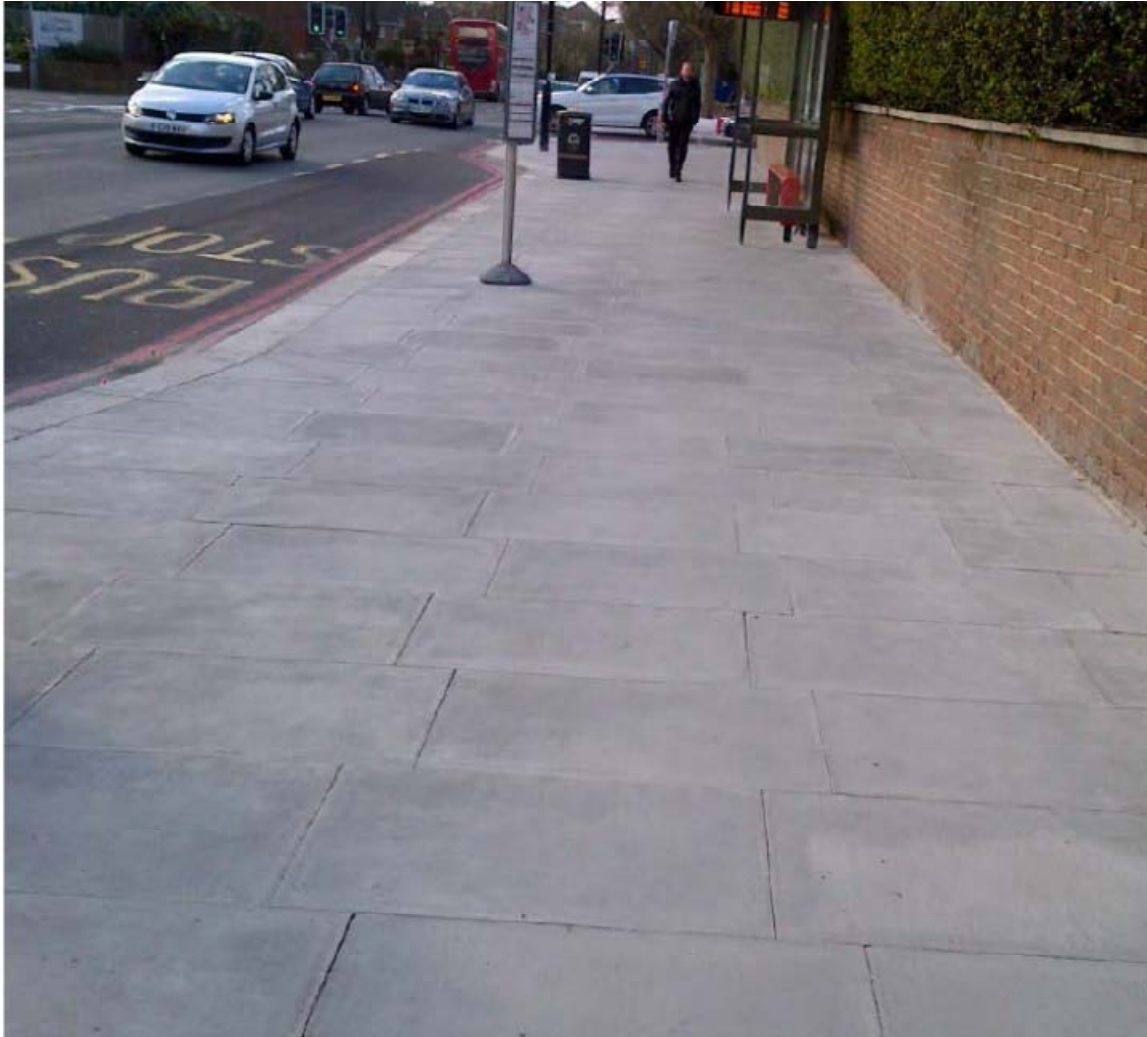
Upper Richmond Road footway works
