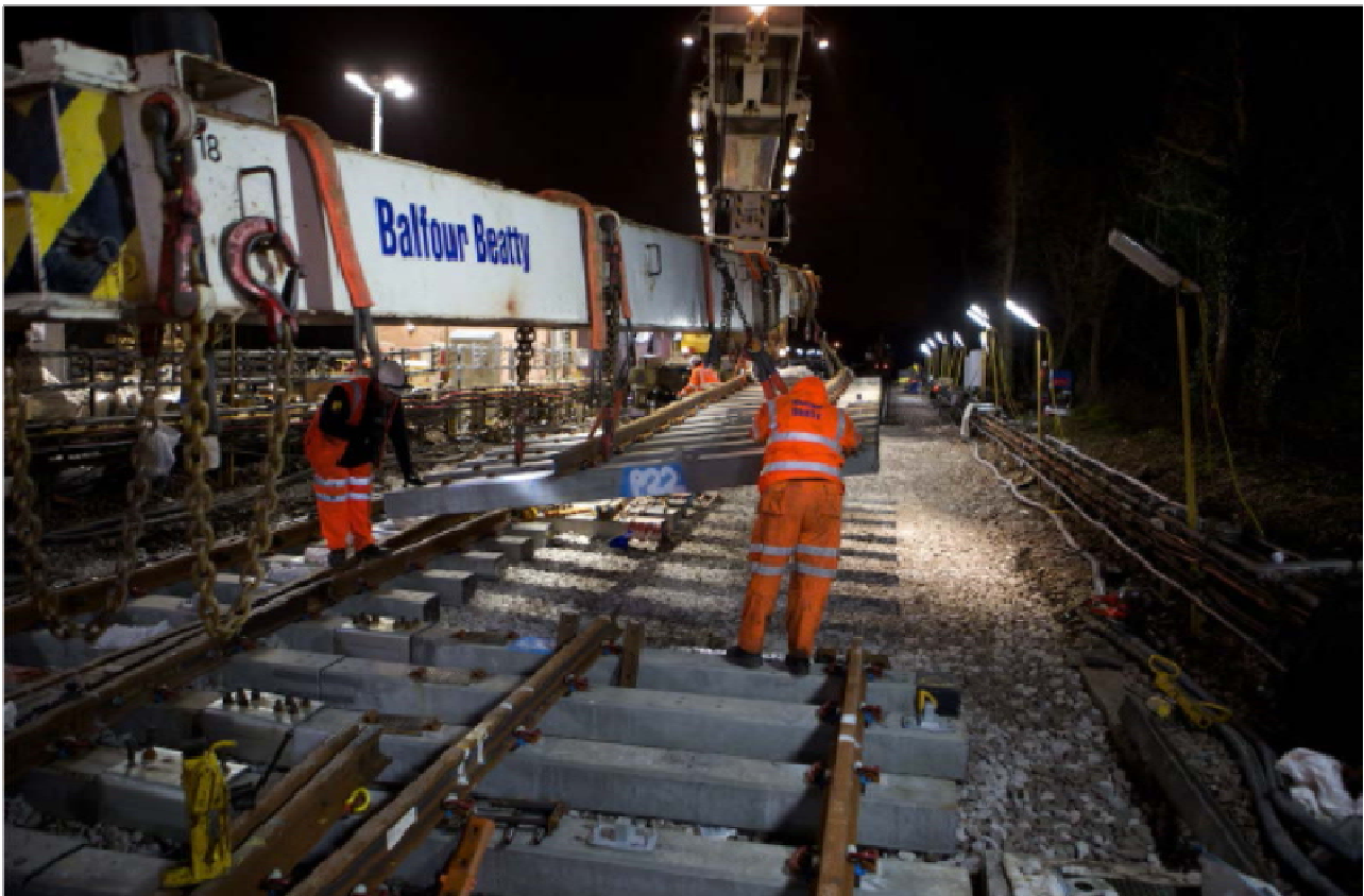
Modular points and crossings installation at Ruislip
