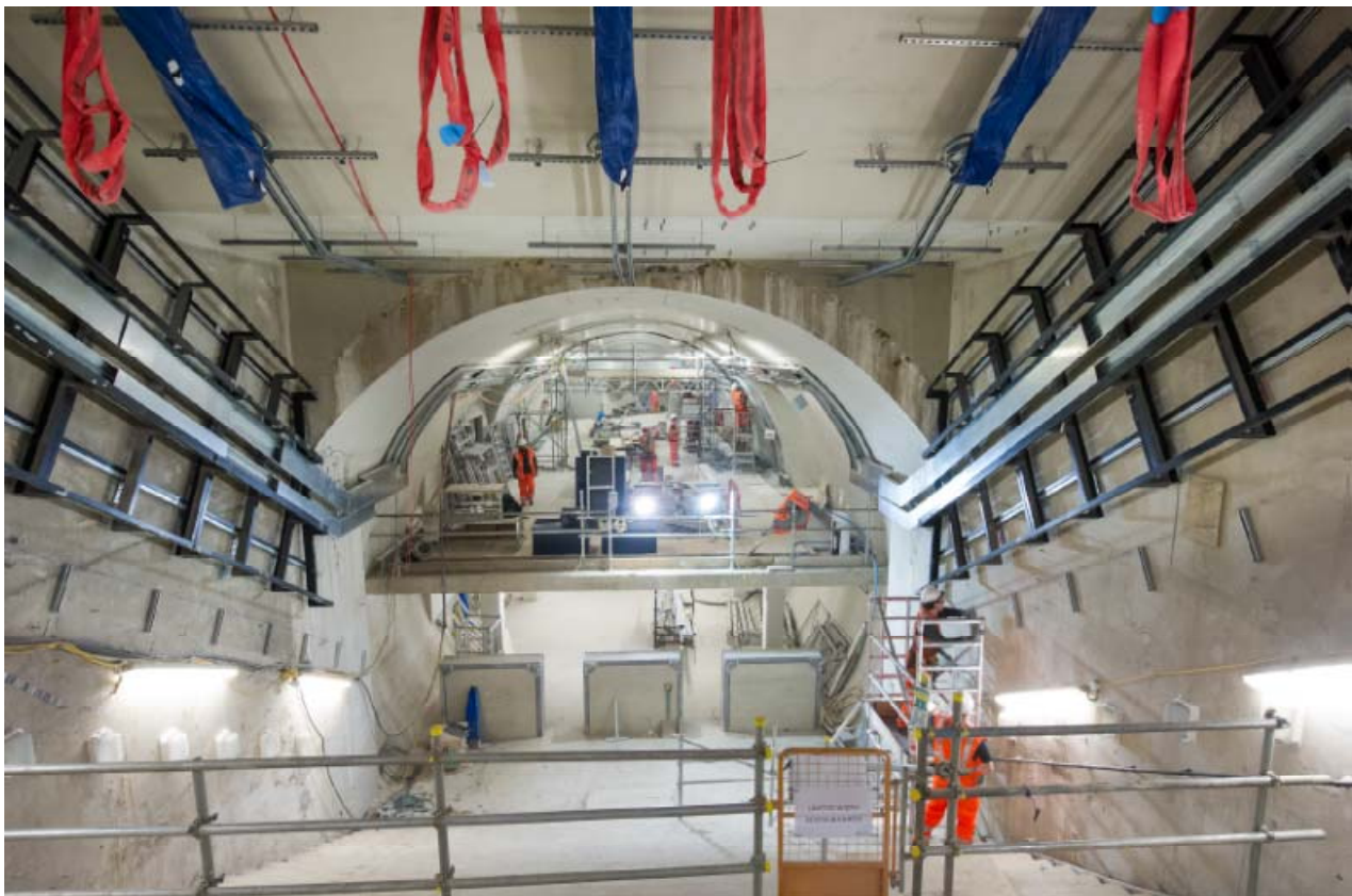
Northern line escalator box for new escalators 7, 8 and 9
