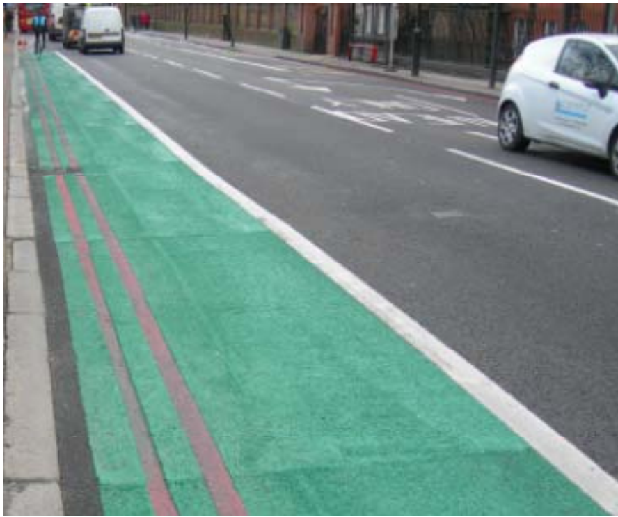
Newly constructed CS5 in use at A202 Camberwell New Road, Eastbound between Brixton Rd and Bolton Crescent
