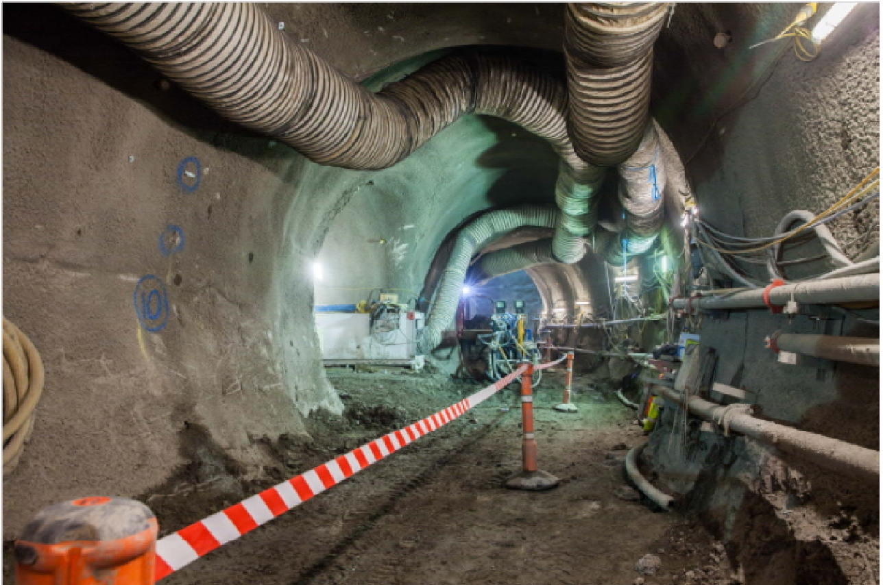
Bond Street tunnelling works
