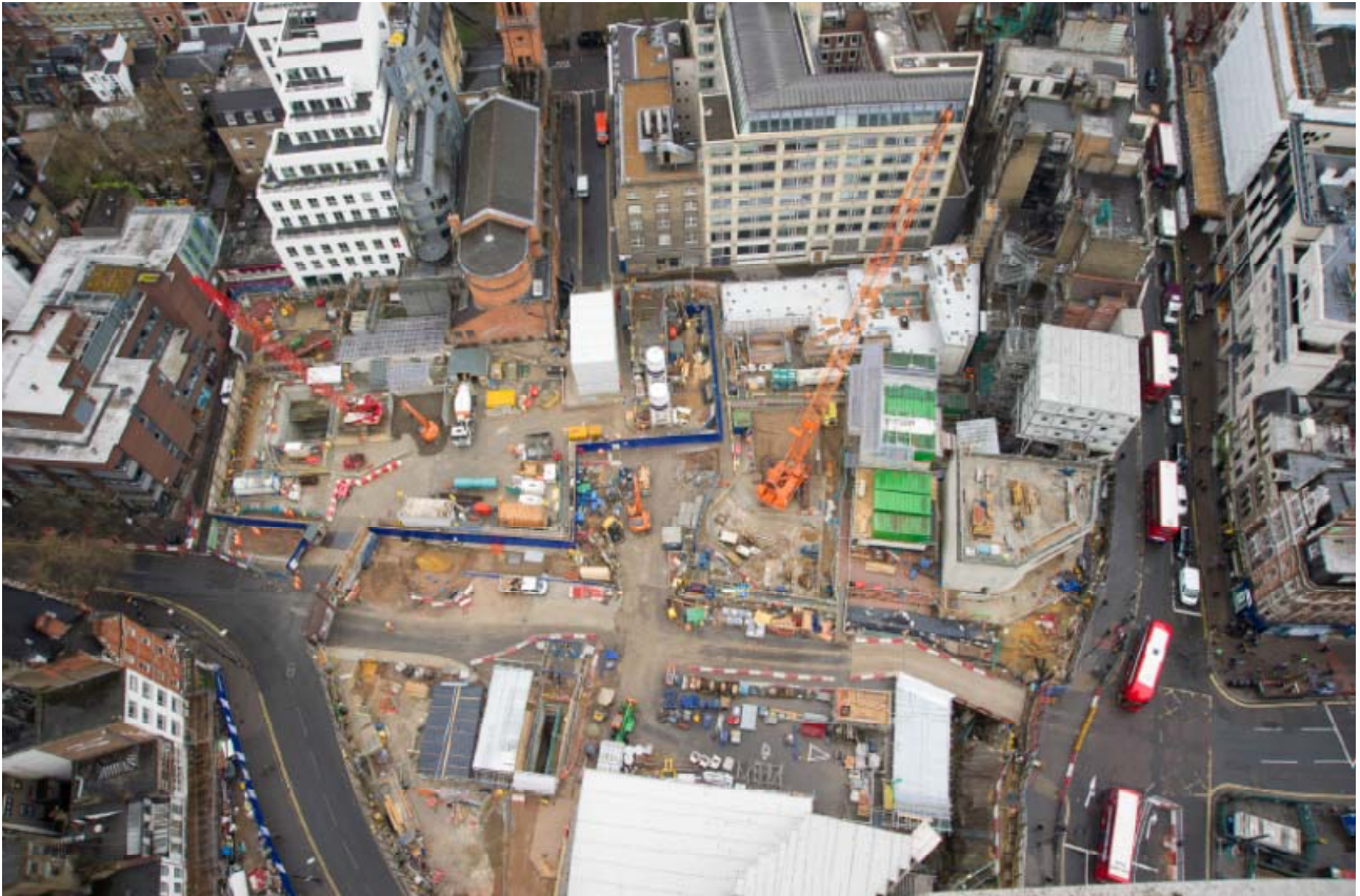
Aerial view of whole site at Tottenham Court Road
