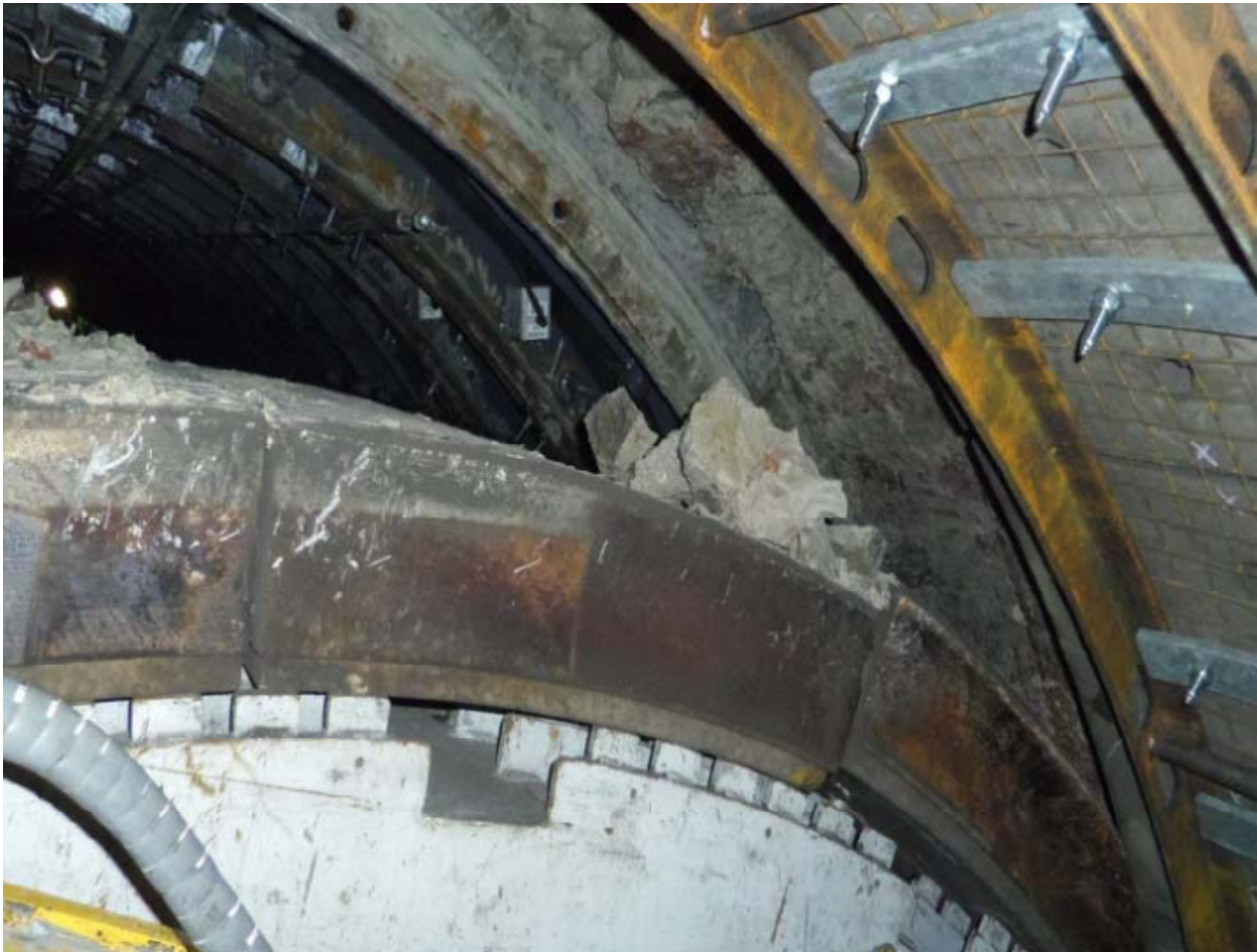
Shoulder tunnel segment being lowered
