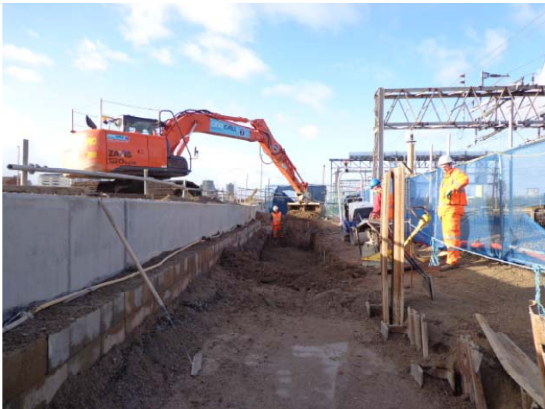
Twin tracking infrastructure works
