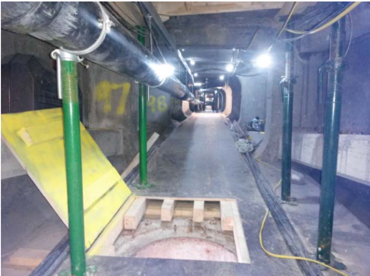
Inside Hammersmith Flyover
